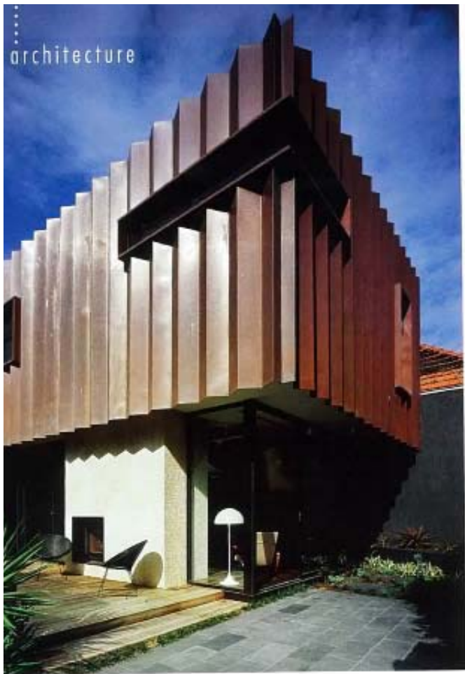
ABOVE: In time, the pleated, copper sheeting cladding – initially coloured a raw pink/orange – will oxidise to a deep brown. TOP RIGHT: The double-sided gas fire (behind the lamp) helps heat the living room and warm the decked, outdoor eating area at the side. PICTURES: SHANNON ACRANH
