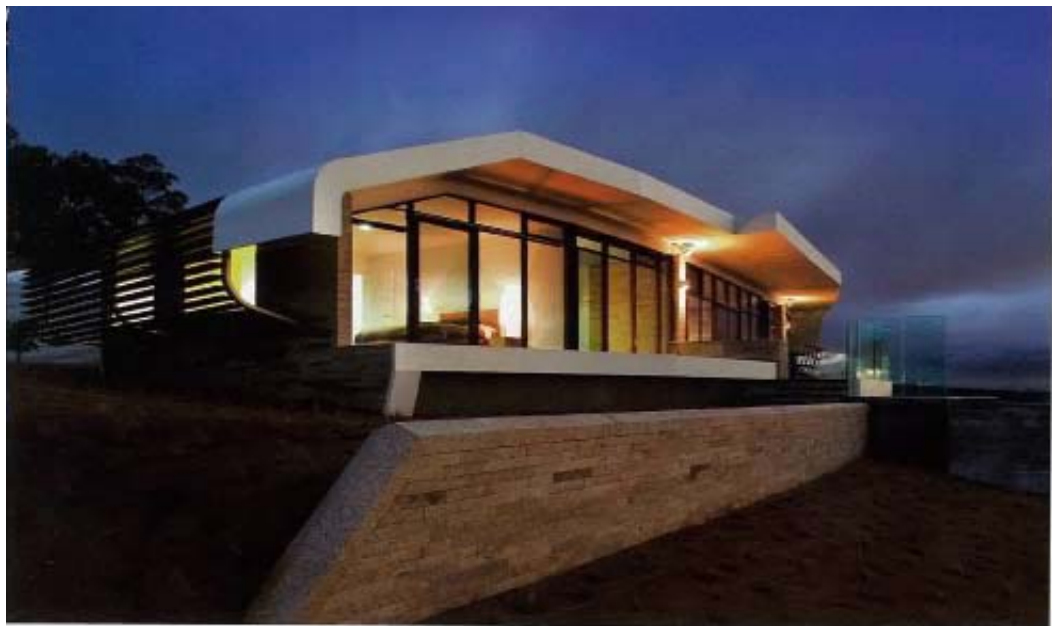
ABOVE: A steel canopy extends over the sweeping northern facade and acts as a temperature control for this house in the Strathbogrie Ranges. LEFT: The windows of the bedrooms are enclosed by curved timber louver screens. PICTURES: JOHN GOULINES
